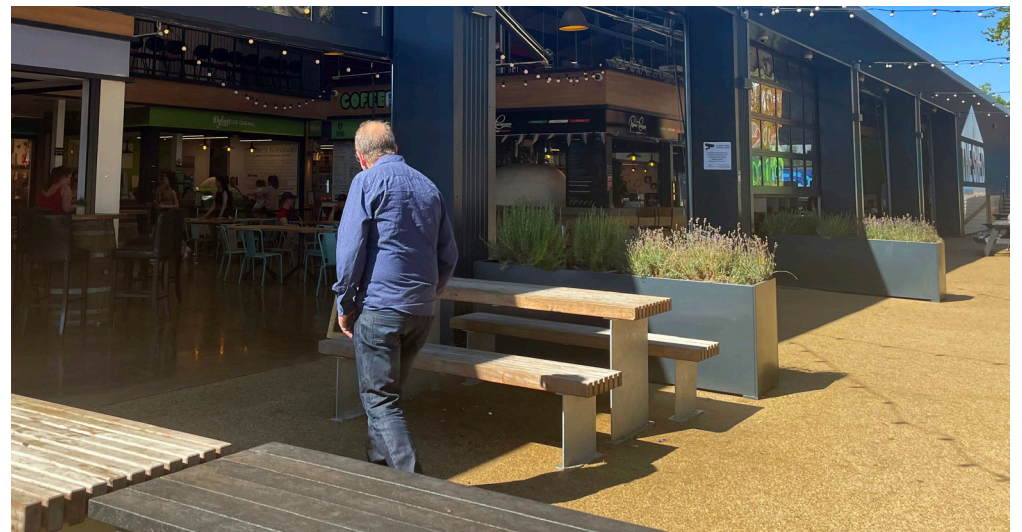
Figures 12 & 13. The Shed in the new community at Whitehill and Borden is an adapted agricultural portal-frame shed with small business units within it. It is home to a number of local, indigenous businesses, is a popular meeting place for residents and an easily recognisable part of the community's identity. (Images EDDC 2021)
